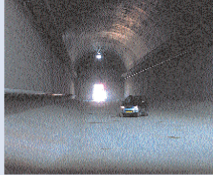
DTT under construction.
